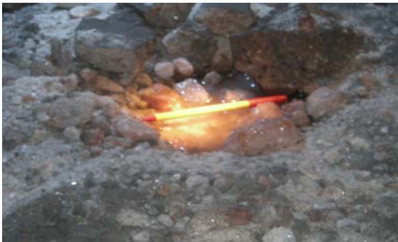
Figure 11: Brine solution on the floor of chamber 46
