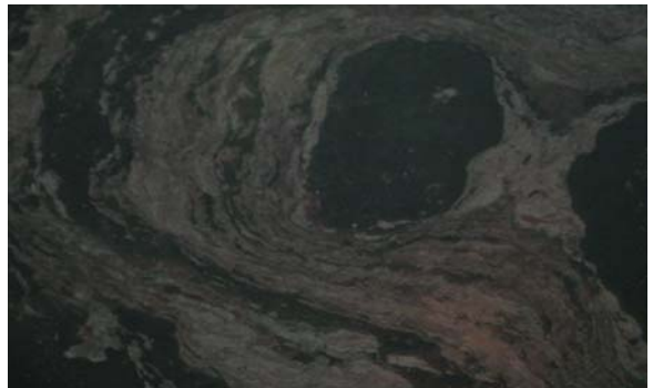
Figure 12: Effects of humidity on the roof of chamber 46 disturbing the salt layers
